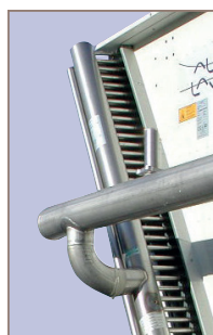
Stainless steel tubing for ammonia application (ANV)
